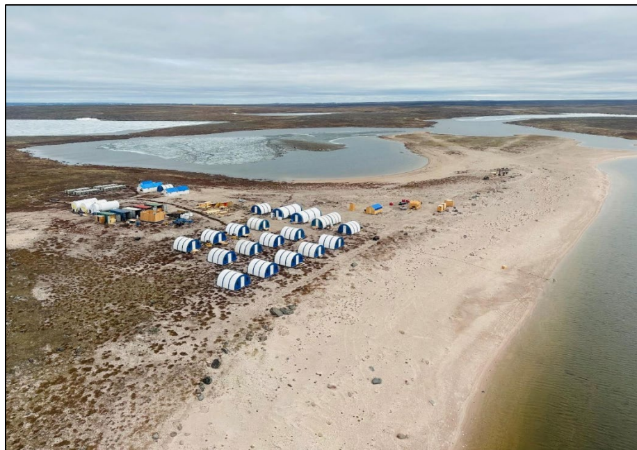
Forum’s newly-constructed 30-person drill camp located on Aberdeen Lake at west end of property
